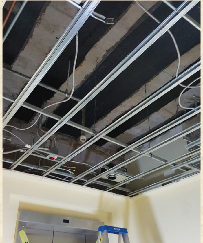
Installation of FRP System above finished elevator lobby
