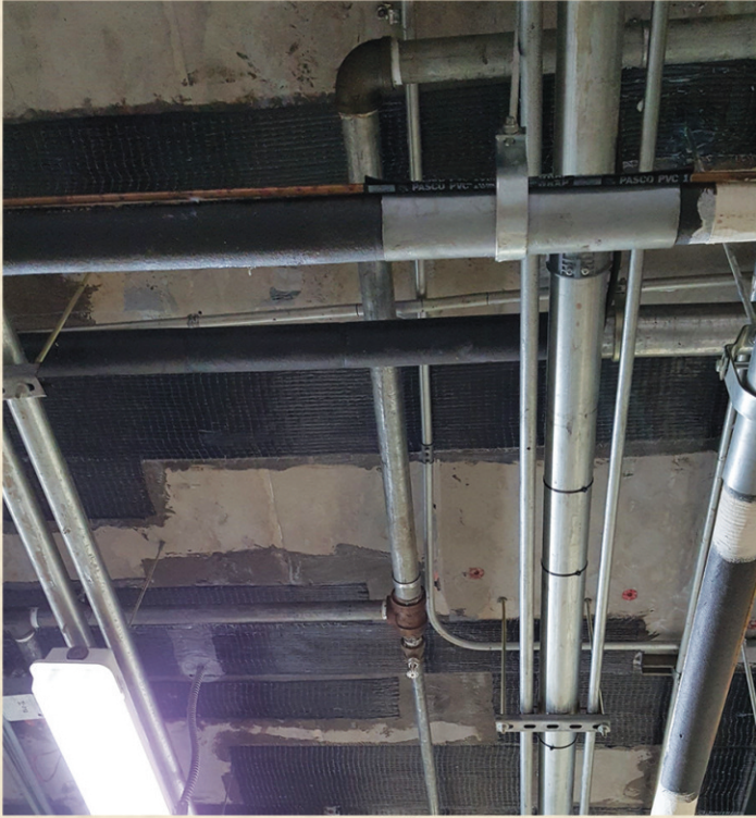
Installation of FRP System through existing MEP
